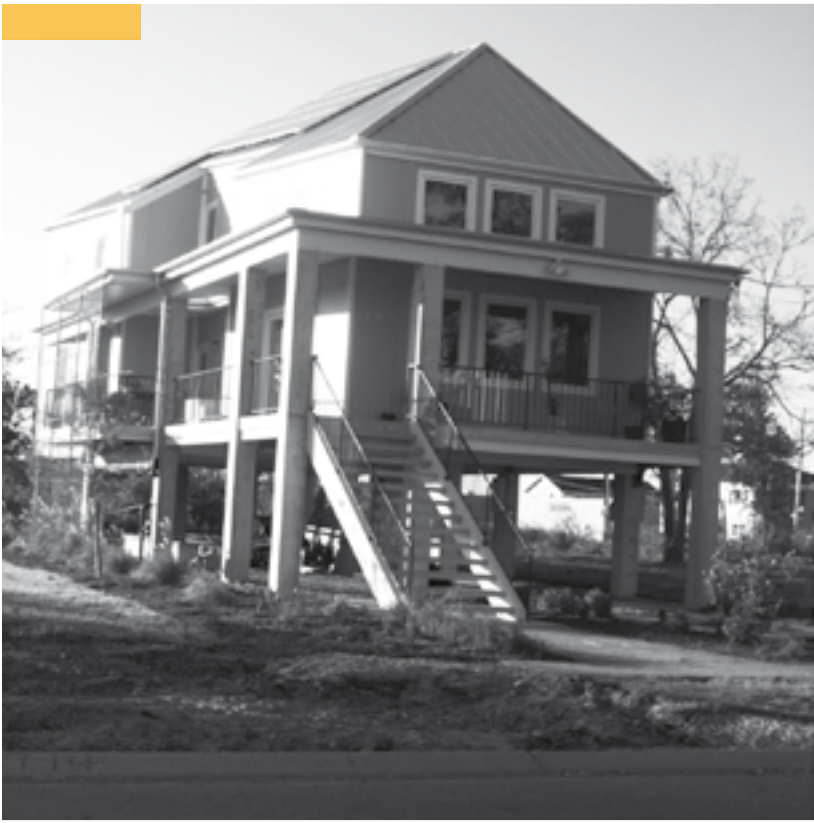
Houses built on 8 feet stilts to avoid flood waters
